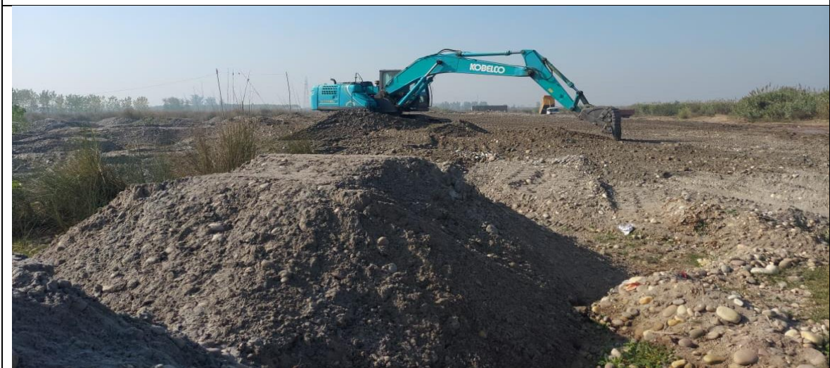
Plate 3- Desilting site of Bari Haveli Ropar
