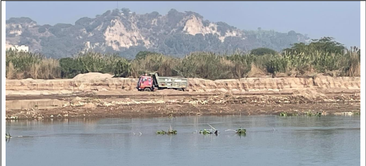
Plate 1- Desilting site of Bari Haveli Ropar
